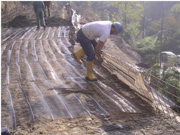
Figure 3c – Positioning of the pre-seeded biomat and of hooks
