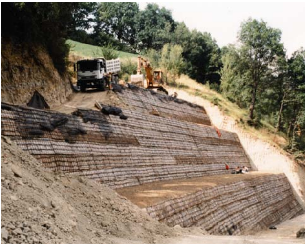
Figure 3e – Wrapping of the portion of geogrid, previously kept outside the formwork
