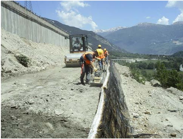
Figure 3d – Soil compaction
