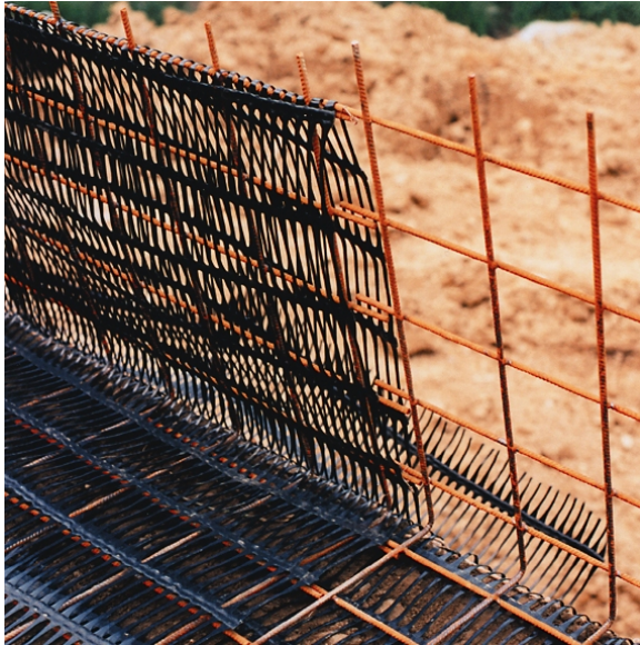
Figure 3b – Positioning of the reinforcing geogrid
